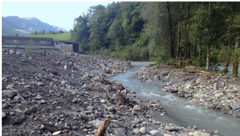
Wet-dry channel with flattened riverbank and planted rootstocks.
