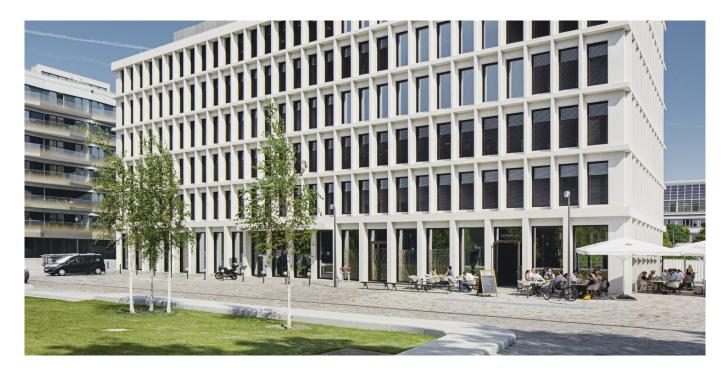
The scope of EBP's planning activities in Germany includes its own new office building in Berlin. The focus of this project was on the seamless and slender façade made of cast-in-situ concrete and the energy-efficient, low-permeability building envelope behind it. The biggest challenge was to enable the construction of the low-permeability building envelope despite the fact that the inner shell and the outer concrete facade would already be in place at the time of the envelope's installation.
