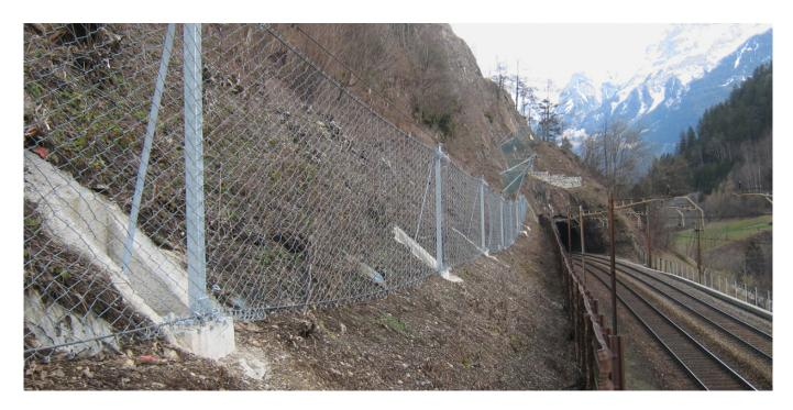
Around 4,700 protective structures currently protect the SBB railway network against rock falls, flooding, avalanches and other natural hazards. Working together with SBB representatives, EBP has developed a concept for a simulation model that calculates the resources that will be necessary to secure the long-term maintenance of these structures.
