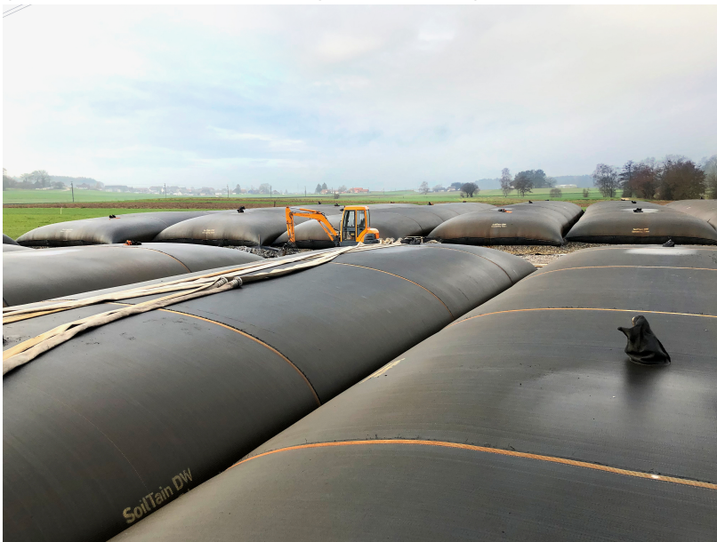
Filled geotubes at the drainage site
