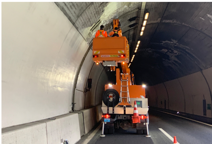
Tunnel condition inspection
