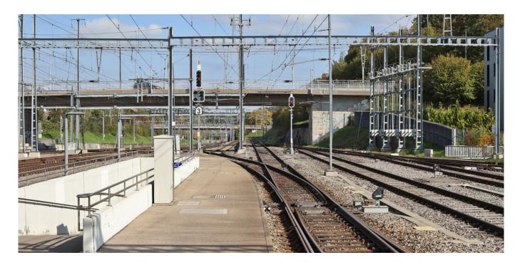
Effretikon Train Station has various shortcoming and does not meet all of the requirements of the Swiss Disabilities Act. By removing the existing track 4, a good solution that meets all the requirements has been found, with a new pedestrian underpass and the widening of the two central platforms. The structural measures require extensive adjustments to the entire station: tracks, platforms, all entrances and the bicycle crossing must be redesigned.
