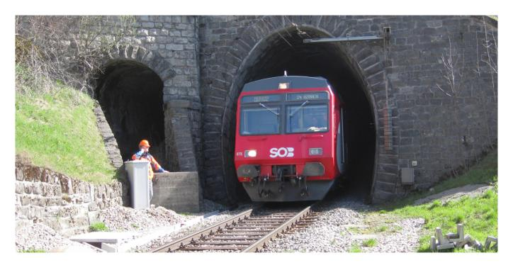
The Swiss South Eastern Railway's single-track Wasserfluh Tunnel, over 100 years old, needed comprehensive repairs and technical re-equipping, and the floor was lowered in places.
